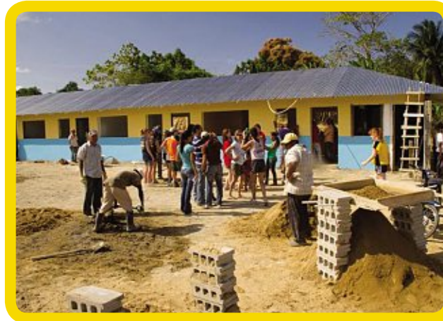
Building a school in the Dominican Republic.
